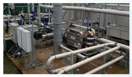
Dwr Cymru commissioned Marches Biogas Ltd to manage the maintenance works and media change of the Parker PpTEK Siloxane Removal System's (SRS) at Afan WwTW and Five Fords WwTW.
